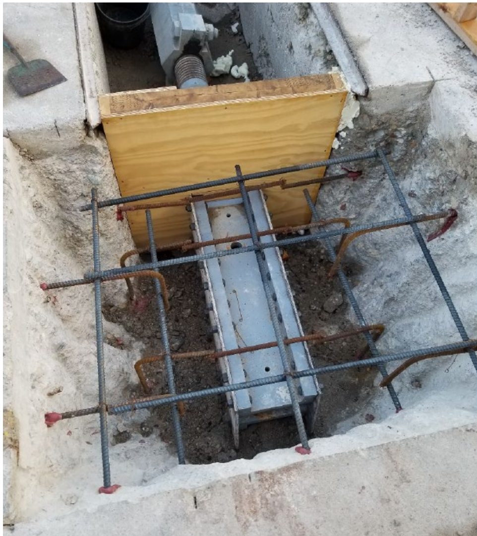
Miter gate anchorage repairs
